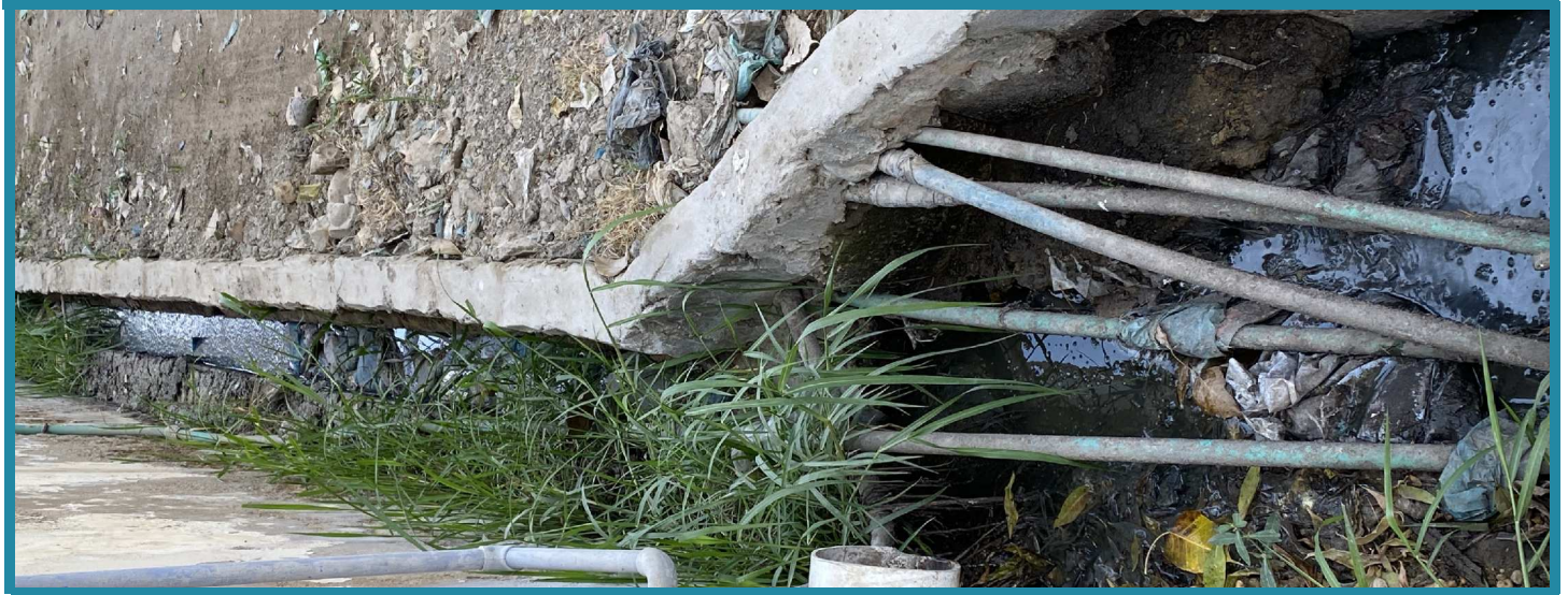
Badin: A city where potable and drainage lines run sid-by-side often intermingling.
