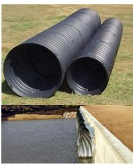
Culverts are commonly used both as cross-drains to relieve drainage of ditches at the roadside, and to pass water under a road at natural drainage and stream crossings. A culvert may be a bridge-like structure designed to allow vehicle or pedestrian traffic to cross over the waterway while allowing adequate passage for the water.
